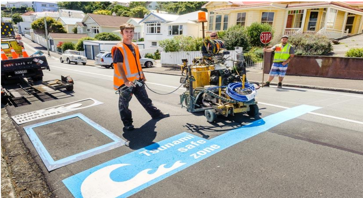
A civic employee in Wellington, New Zealand, paints a sign with a wide blue line on pavement crossing the street. The sign includes a graphic of a tsunami wave and the words “Tsunami Safe Zone”. (Photo courtesy of Mark Coote: www.markcoote.com )
