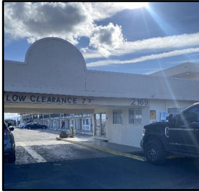
Los Banos Emergency Housing
