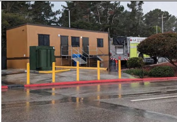
Modular trailer "fire station" at airport
