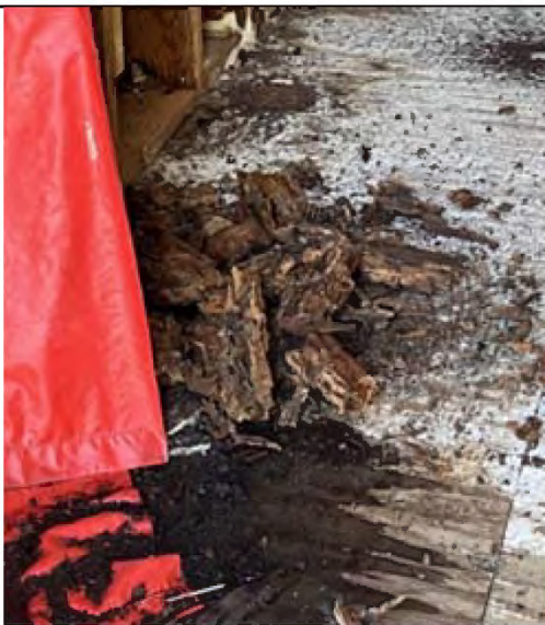
View inside abandoned training tower
