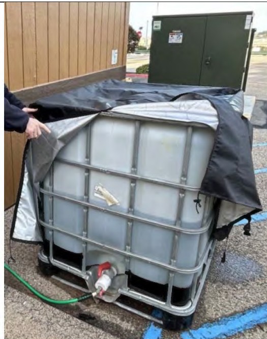
Non-potable water supply
