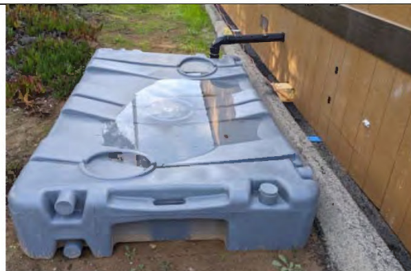
Septic system for modular trailer
