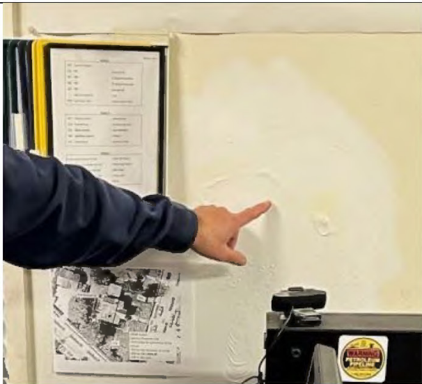
Bubbling paint after two weeks
