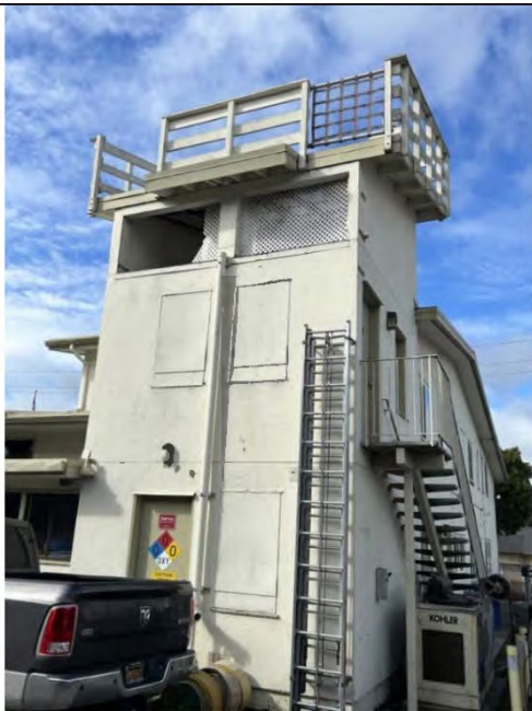
Abandoned training tower
