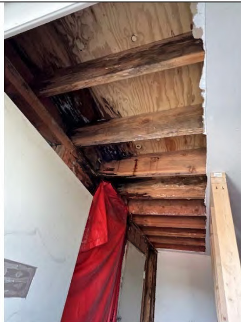
View inside abandoned training tower
