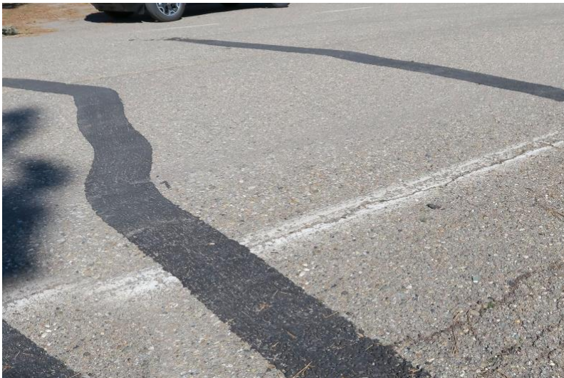
Photo: Crack sealing on Meadowbrook Loop, Chester, CA. 2026
