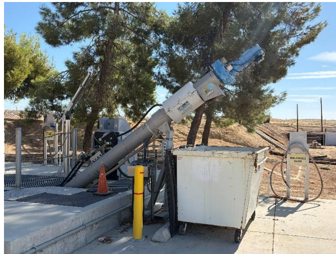
Auger located at wastewater treatment plant Picture taken by Grand Jury
