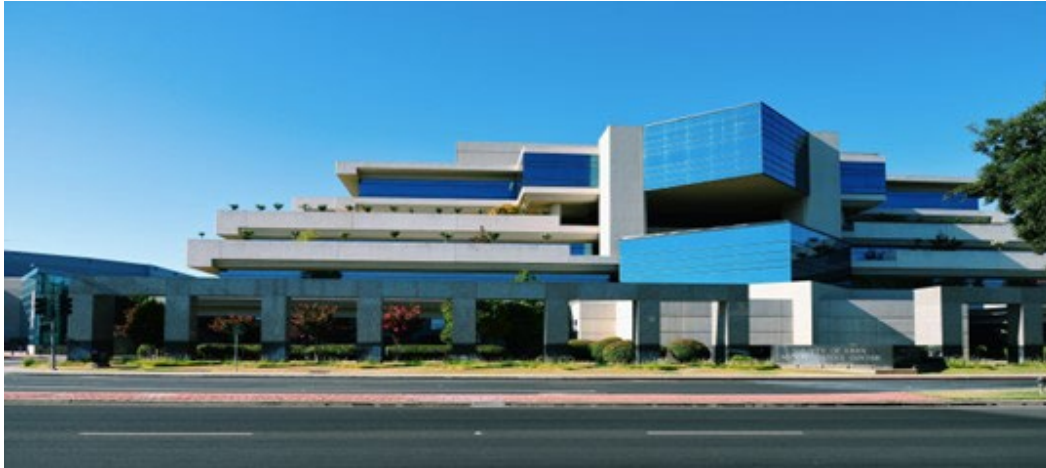
Kern County Administration Building Photo from the Kern County website
