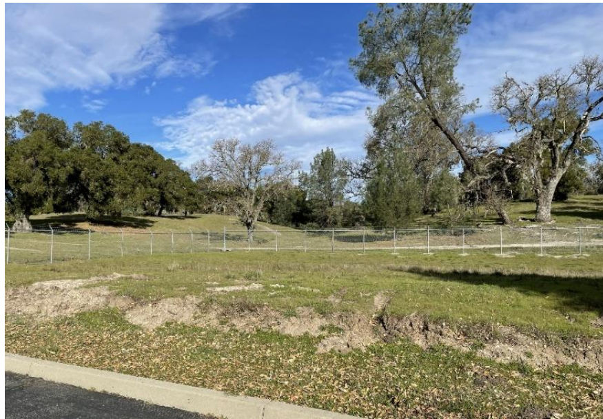
Photo of new fencing around expanded area.
