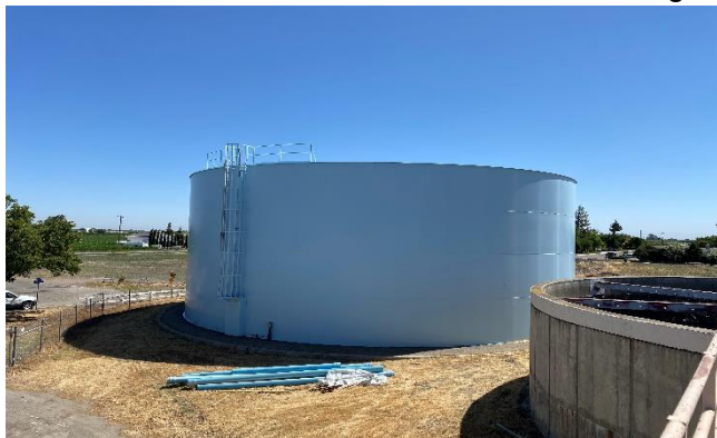
Figure #4: Existing ground level storage tank.
