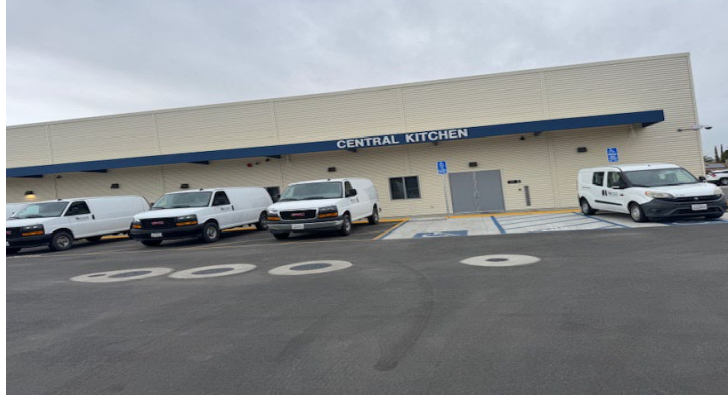
Kern County Superintendent of Schools Central Kitchen Photo Taken by Grand Jury
