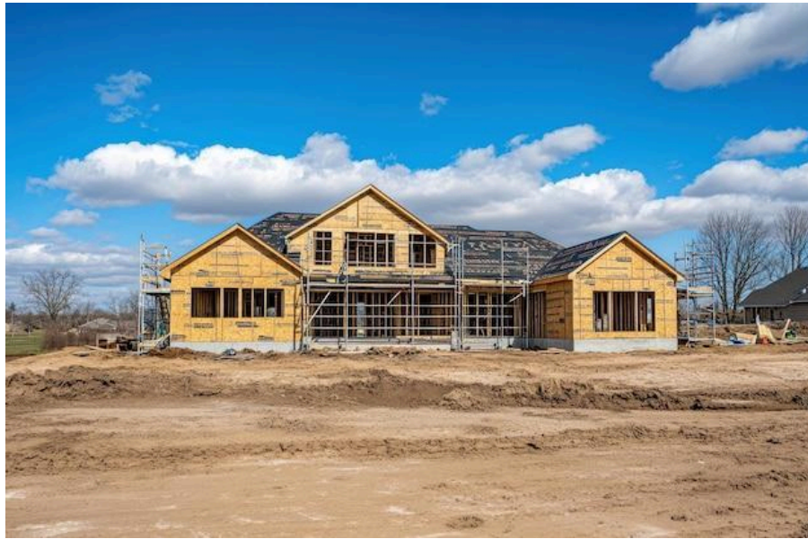
Picture of a home under construction
