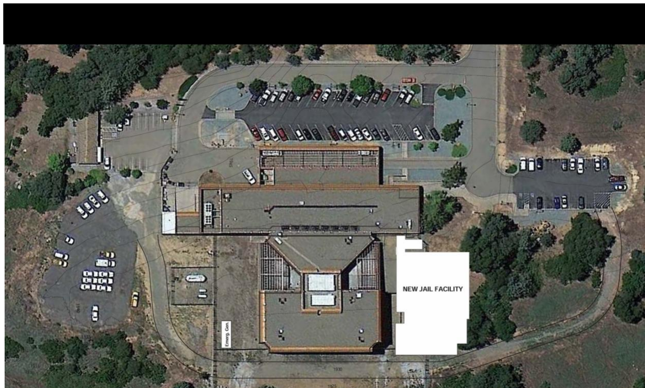
El Dorado County Jail – Placerville Facility Expansion Project
